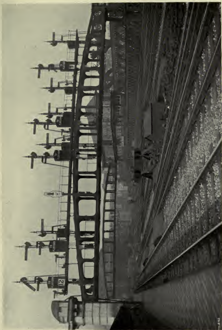
SIGNALS, GLASGOW CENTRAL STATION.
